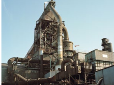
2. Mineral weighing—blast furnace
